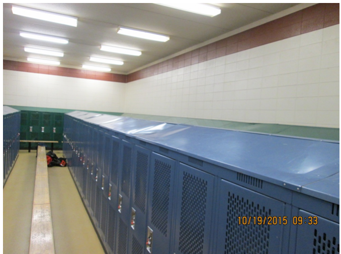
The Locker Rooms are generally in good condition. There is damage evident on the slope tops on some of the lockers and the finishes on wood benches are worn down.
